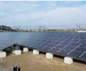
The solar power installation No.1 at the Shiga Plant
