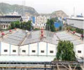
Solar power generation in Bhiwadi, India
