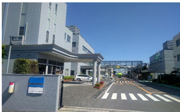
Installed at Tokyo Plant (Noda city, Chiba)
